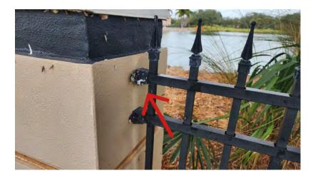
Nine anchors are missing and need to be replaced.
